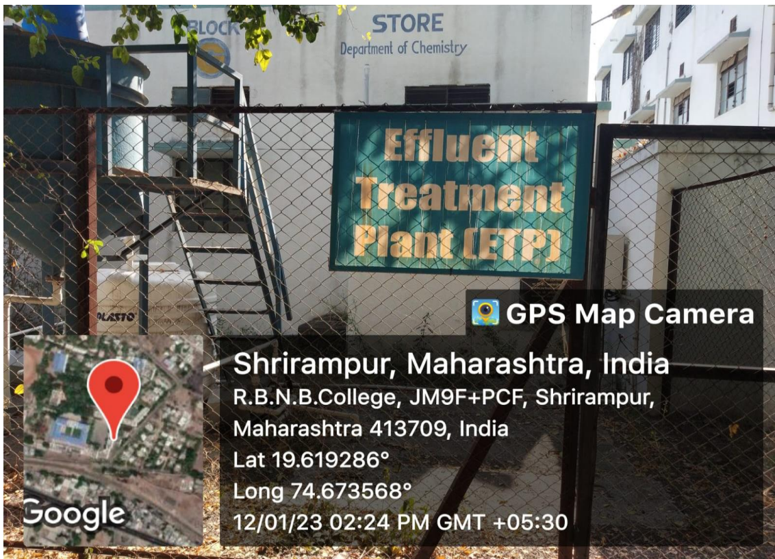
Effluent Treatment Plant (ETP) for water recycling
